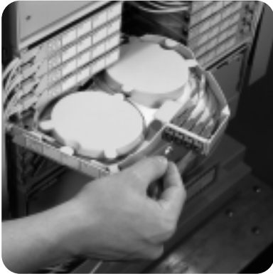
Figure 3: Jumper is connected
