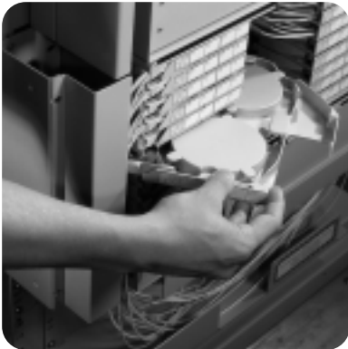
Figure 1: Drawer rotates open on hinge
