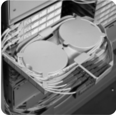
Figure 4: Jumper is routed and stored by looping around spools
