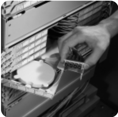
Figure 2: Pigtail routes and connects using 'S' loop
